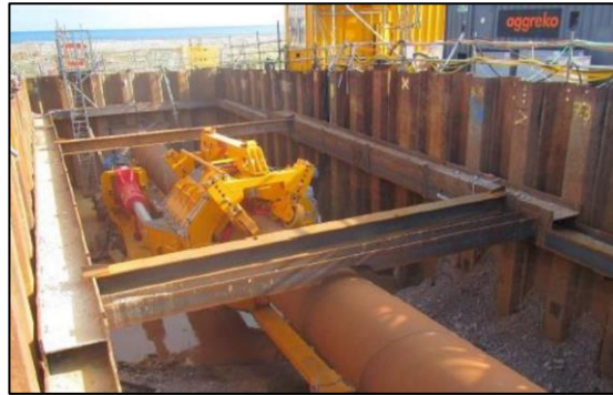
Figure 2: Temporary cofferdam installed on a beach (brown sheet metal), with trenchless technique equipment inside of it. [Plate 3.4 of AS-024]
